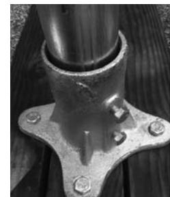
3. Take the post bottom (the end without threaded holes) **and insert into decorative base top** and down into the cup bolting flange.
